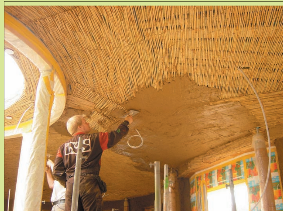
First layer of clay applied on reed mat
