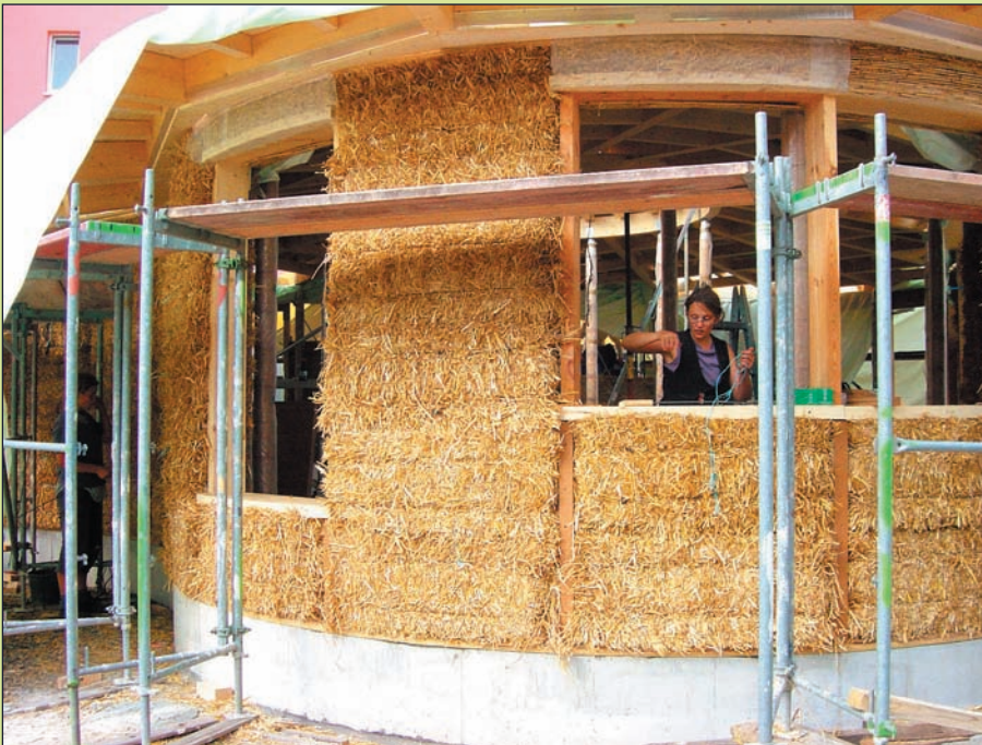
Straw-bale wall provides high insulation
