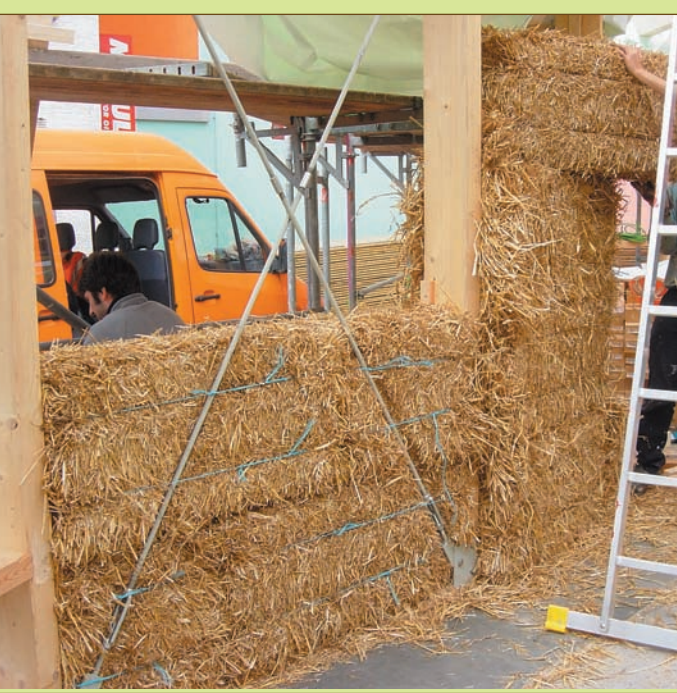
Reinforcement in strawbale wall
