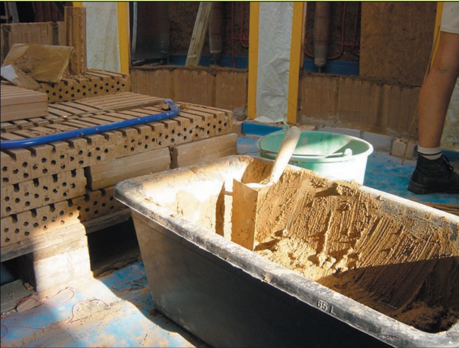
Adobe bricks are used for the interior walls
