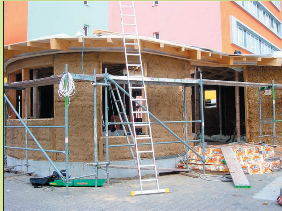
First layer of clay on strawbale wall
